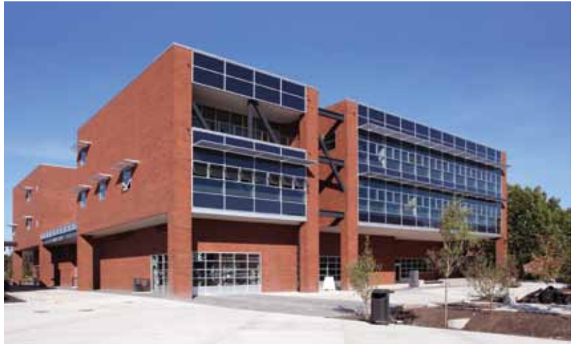
Bellingham Technical College's new Campus Center is designed to be energy efficient and will offer high-quality, industry-standard learning environments for students, according to school officials. Outdoor sitting areas with native-plant gardens and an outdoor sculpture by artist Ilan Averbuch are set to be installed by December. Photo courtesy of BTC
